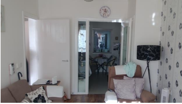
Figure 2: Living room with glazed partitions to kitchen for borrowed light, Case Study 3.
